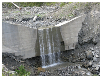
Scouring phenomenon downstream a check dam. Saint Antoine torrent, France, 2014. Source: [Chahrouh et al., 2021]
