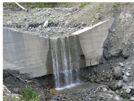
Scouring phenomenon downstream a check dam. Saint Antoine torrent, France, 2014. Source: " INRAE/ETNA. [Chahrouh et al., 2021]
